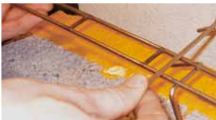
BI-binder legges rundt fugearmeringen
